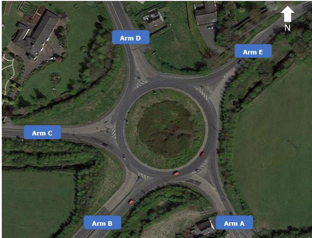
Figure 10.38. Junction 5 Nine Mile Stone Roundabout.
